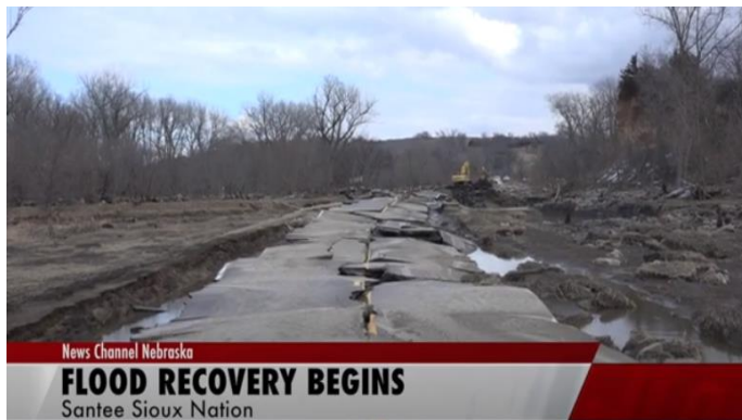
Highway 12 at the western edge of the Santee Sioux Reservation. Road completely destroyed by the flooding of 2019.
