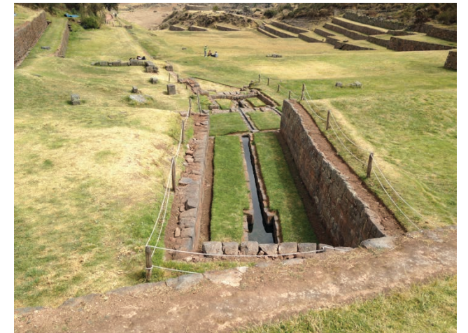
Incan irrigation system
