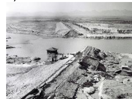
Banqiao dam failure; China, 1975
